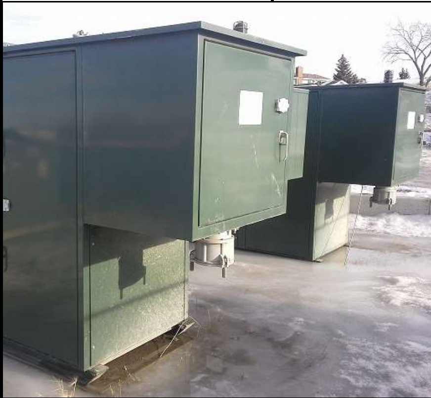
Shown Above: MCS Manufactured 15kV, 600A Female Equipment Mount Couplers in service
